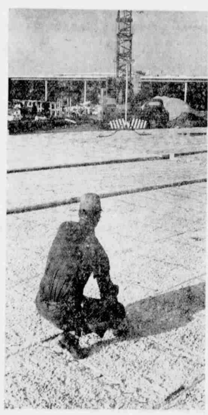
South Mecklenburg High School, now under construction, definitely will not be a fire trap. Here, a construction employee works on a fireproof concrete slab floor in one of the new buildings, expected to be completed when school opens in the fall.
