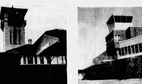
SOUTHERN STATION . . . "practically ready to fall down."
