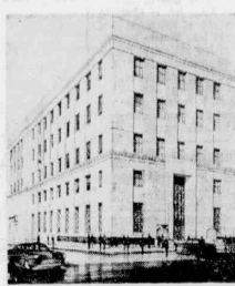
Federal Reserve Bank in Charlotte
