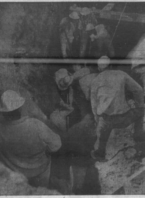
RESCUE ATTEMPT —Members of rescue crew work to free Alfredo Duran, 25, trapped under 30-ton foundation of razed house which dropped on him in ditch. Times photo
