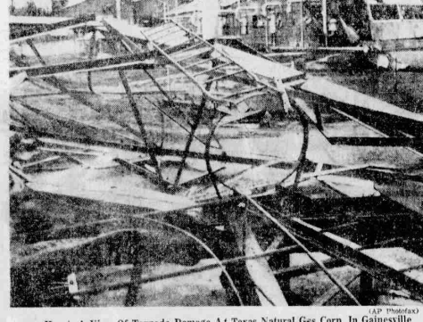
Here's A View Of Tornado Damage At Texas Natural Gas Corp. In Gainesville
