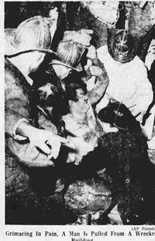
Grimacing In Pain, A Man Is Pulled From A Wrecked Building
