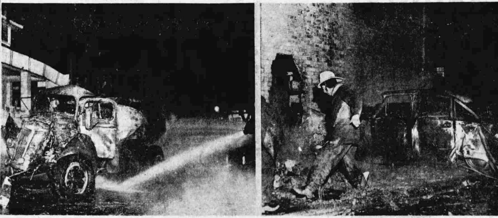
Firemen Hose Death-Trap Tanker At Left, While Others Check Ruined Building And Auto At Spectacular Pre-Dawn Blaze
