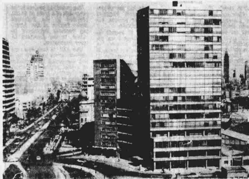
Great Glass And Steel Skyscrapers Are Symbols Of New Era Of Progress
