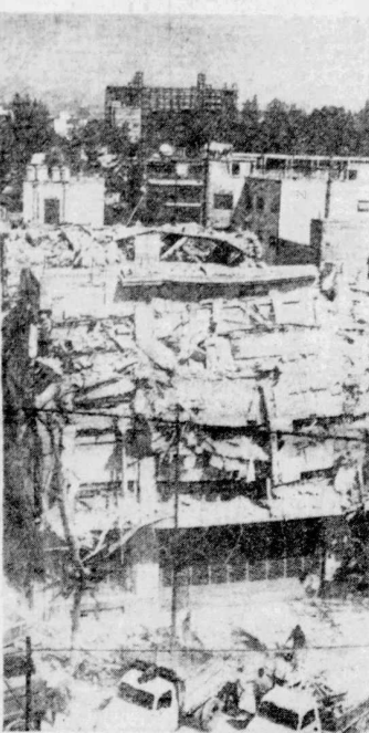
Four-Story Building Collapses During Earthquake
