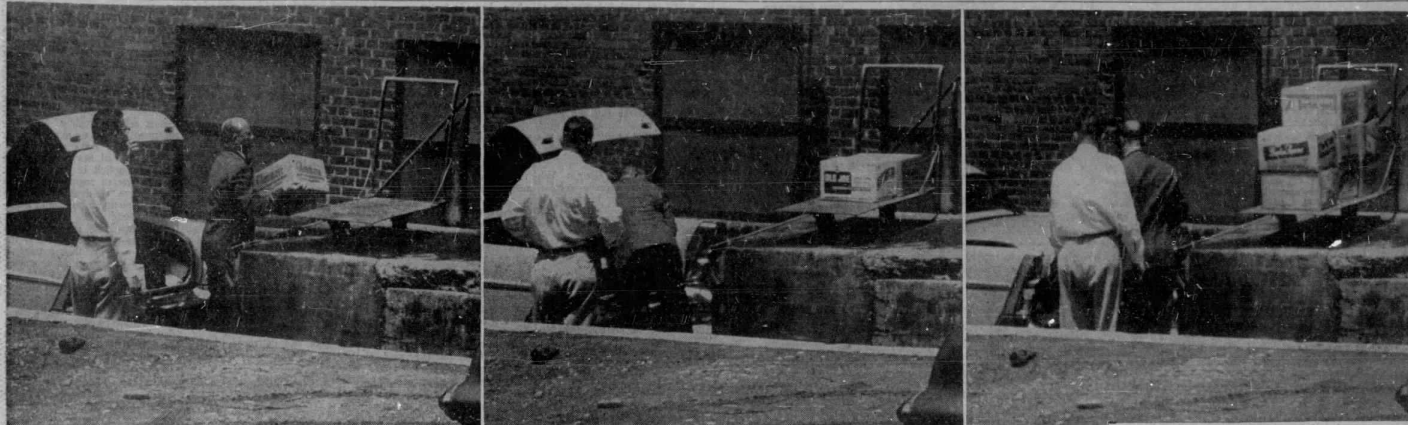
UNLOADING BEGINS, KELLY WATCHING.
