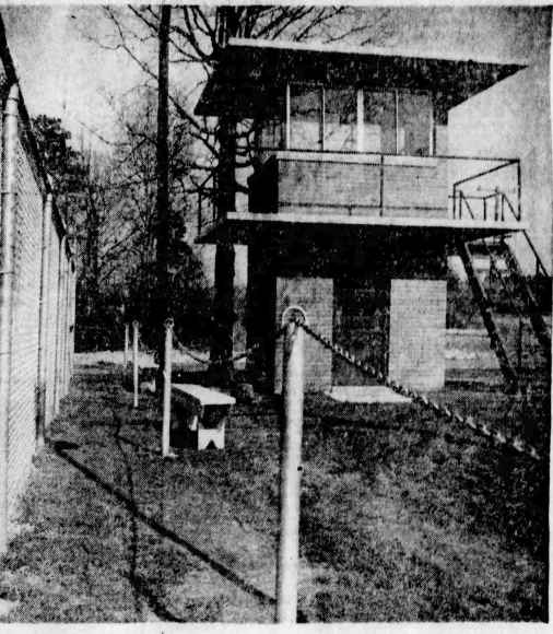
THERE ARE no guards in this guardhouse on the roads or in a stone quarry nearby. When the guards do use the tower, they carry only pistols and do not carry arms to fire at prisoners. Huntersville is a camp for misdemeanor offenders who cannot be shot while in flight.
