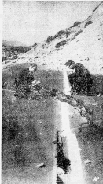
FISSURES CAUSED BY quake are inspected by San Francisco reporters. This highway was blocked by a slide also caused by the tremors.
