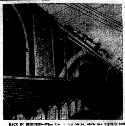
BACK IN BUSINESS—When the Germans retreated in 1944, they destroyed many French bridges, among them this railroad bridge at Nogent Sur Marne, which was originally built in 1855. Here the bridge is being tested by several locomotives. The test successful, bridge was opened to traffic.
